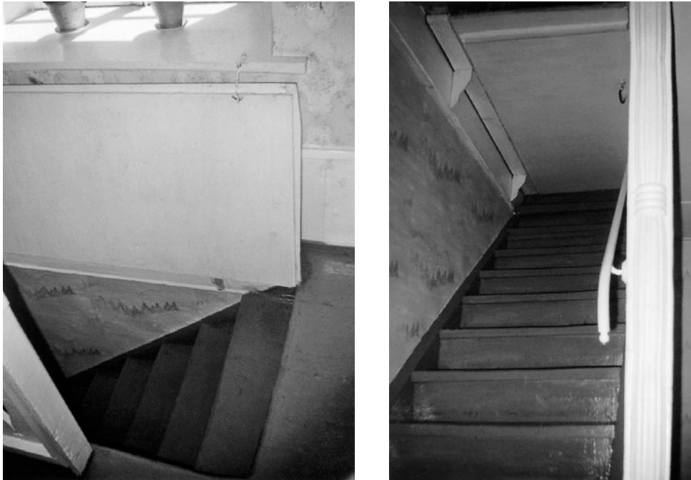
Fig. 9 Staircases pore with the wooden cover <<gabanq>>
