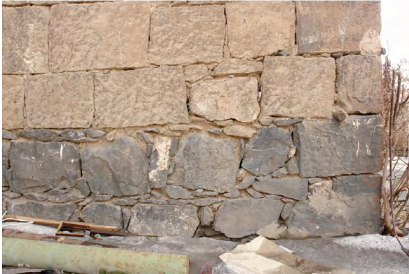
Fig. 5 The foundations are mainly from basalt and mud brick
