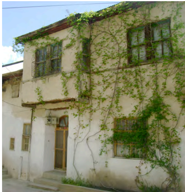
Fig. 4 Traditional residential house in Old Arabkir (Turkey)
