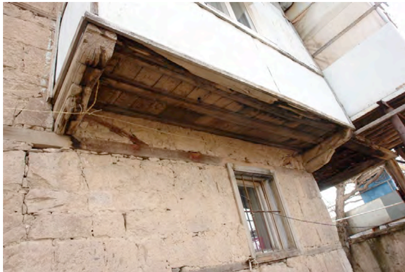
Fig. 6 Special blocks have been made, which could simply move horizontally in case of seismic activity.
